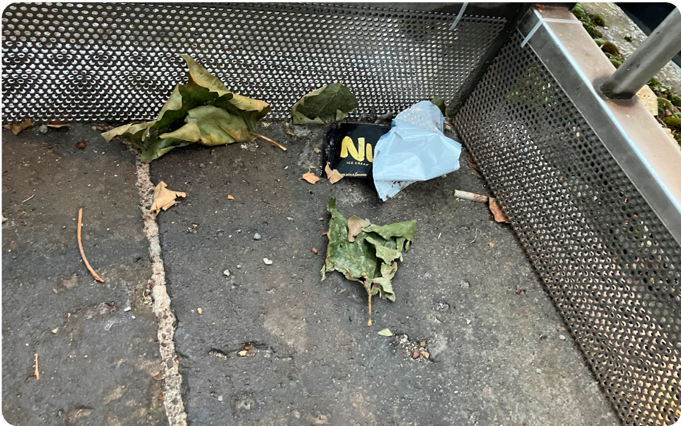
Fig. 5 K.R.A.K.E. Trashstopper installed at the riverfront promenade in Cologne to prevent litter from being washed or blown into the Rhine. Photo: K.R.A.K.E. e.V., used with permission.
