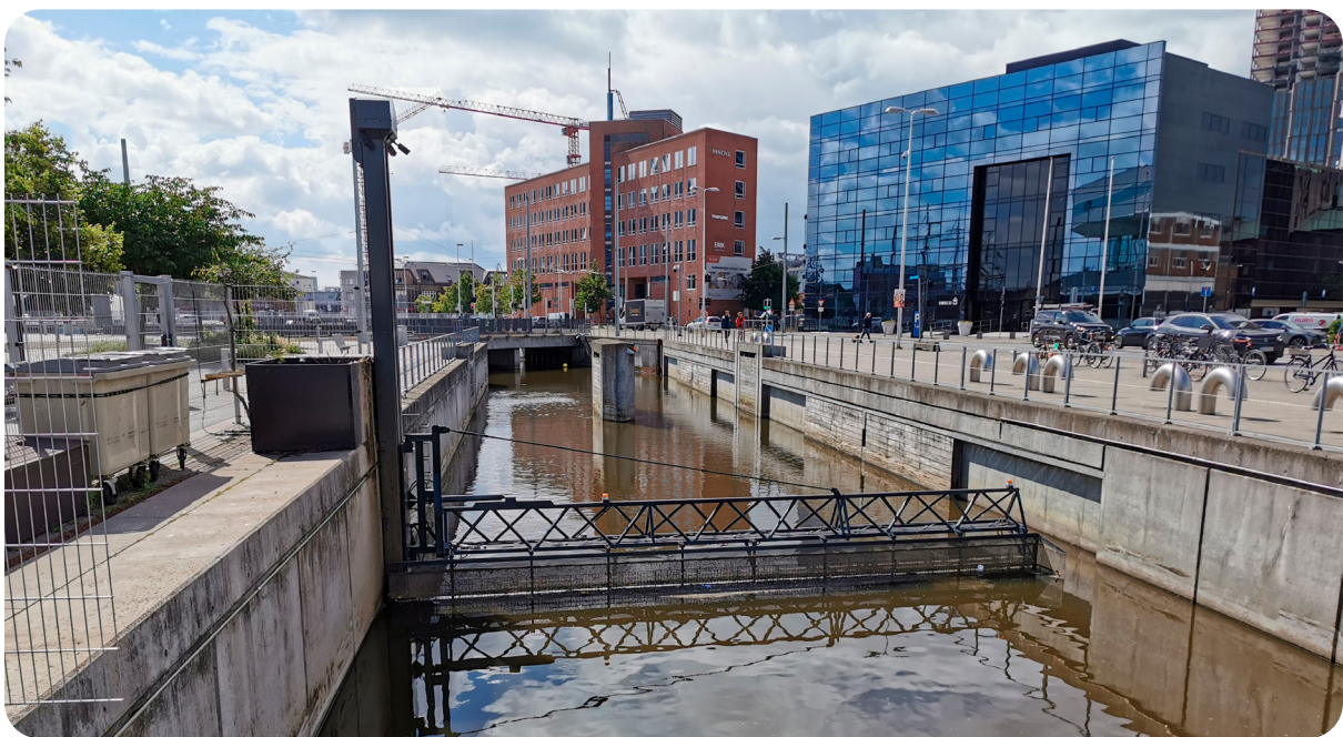
Fig. 6 SeaProtectorOne installed in the Aarhus River, Denmark. The device spans most of the channel width and intercepts floating macro-litter close to the river mouth before discharge into Aarhus Harbour and Aarhus Bay.
